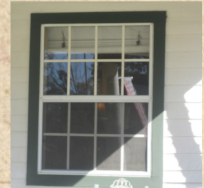
Vinyl window with simulated divided lites incompatible with Victorian architecture
