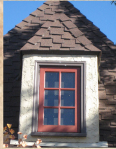
Compatible dormer vent conversion to casement window
