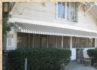
Inappropriate infilled porch features incompatible aluminum windows and awning
