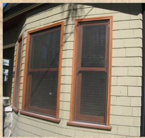
Compatible window replacement for Victorian cottage
